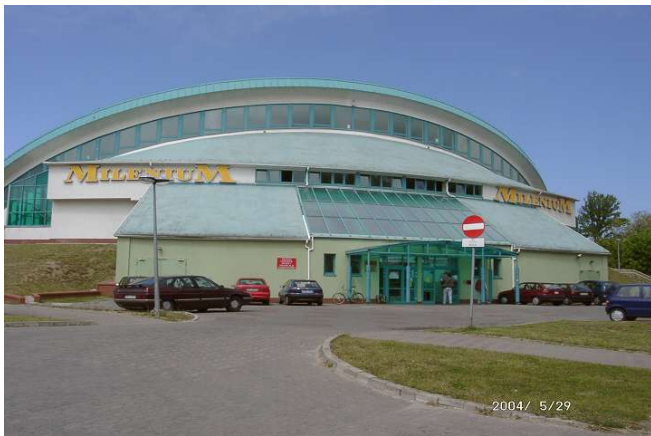
Wettkampfhalle (Hall-Milenium) in Kohlberg
